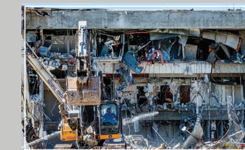
Demolition of Mabel Lee Hall
